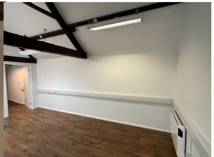
North Wall Internal
