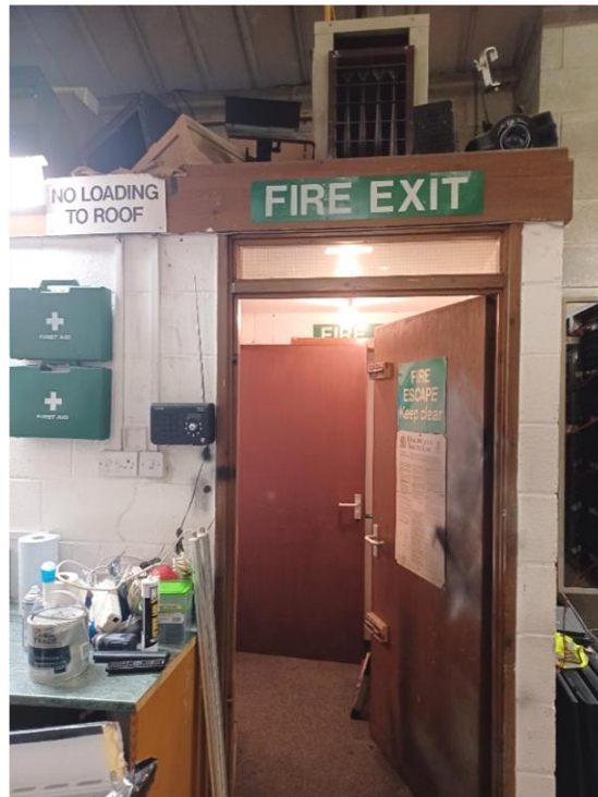
Door to WC
